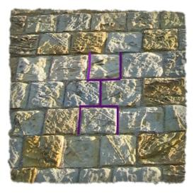
other masons how to cut and set the stone blocks in place using the Norman method of "half-bonding". Today, we wouldn't look twice at a brick wall built that way but the technique adds great strength to a building and ensures that cracks don't appear along weak spots. The great regularity of the stonework on Markinch tower is exceptional and this was the result of imported techniques designed for both strength and speed of construction. It was at its time very much state-of-theart.
